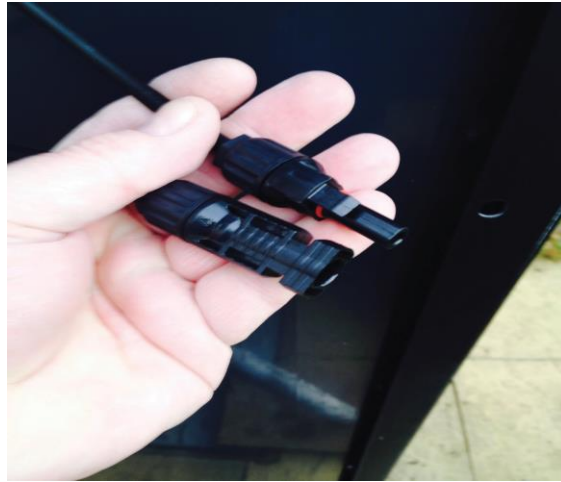
Figure 6.24 DC panel connections
