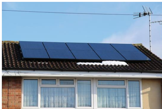
Figure 6.26 A 4kW array of PV panels (ten front and six more at the back)
